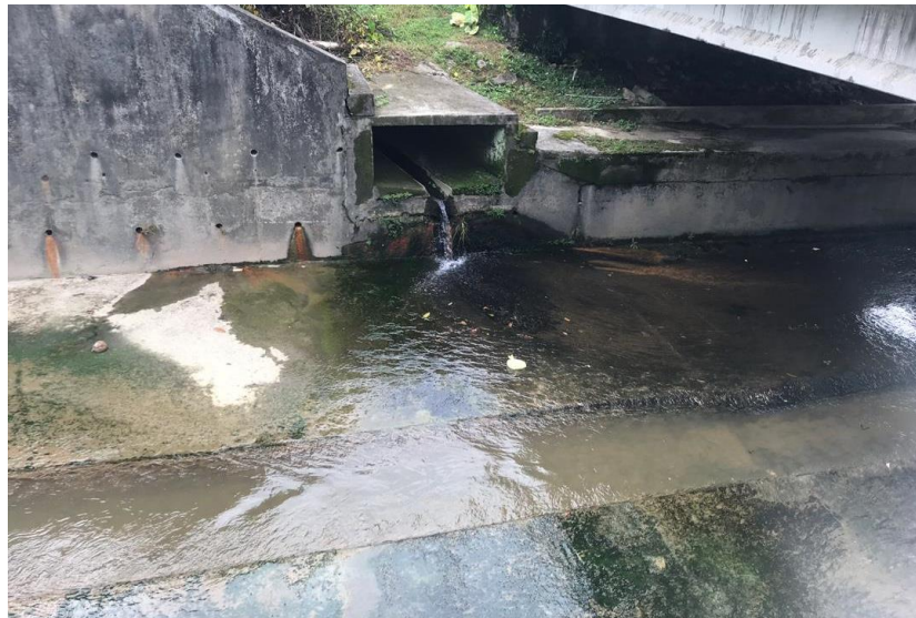
Figure 3. Environmental condition of W2
