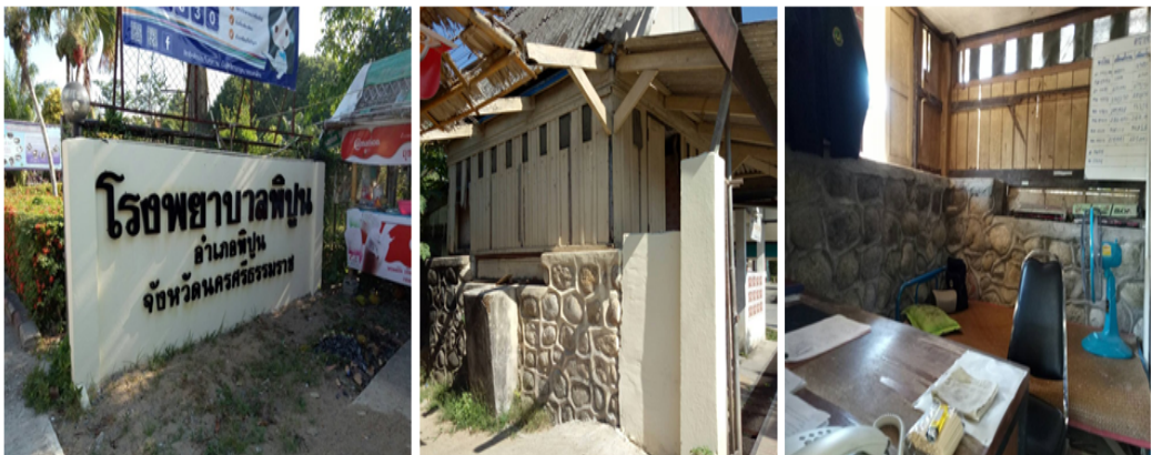
Figure 3: Phipun Hospital, a Former Military Fort is Now Used as an Office for Security Guards
